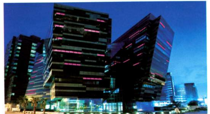
Al Hitmi Office Building, © emdelight GmbH
